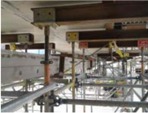
Bagn bru - Redesign of formwork trolley. Prefabrication and installation. Also included design, prefabrication and installation of formwork cassettes.
