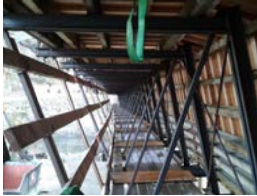
Bagn bru - Redesign of formwork trolley. Prefabrication and installation. Also included design, prefabrication and installation of formwork cassettes.
