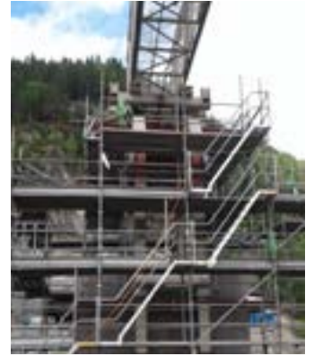
Bagn bru - Redesign of formwork trolley. Prefabrication and installation. Also included design, prefabrication and installation of formwork cassettes.
